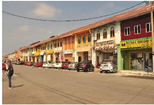
Figure 4: Building facade condition in Pekan Rembau
